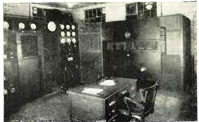
THE R.F. PORTION OF THE TRANSMITTER EQUIPMENT
