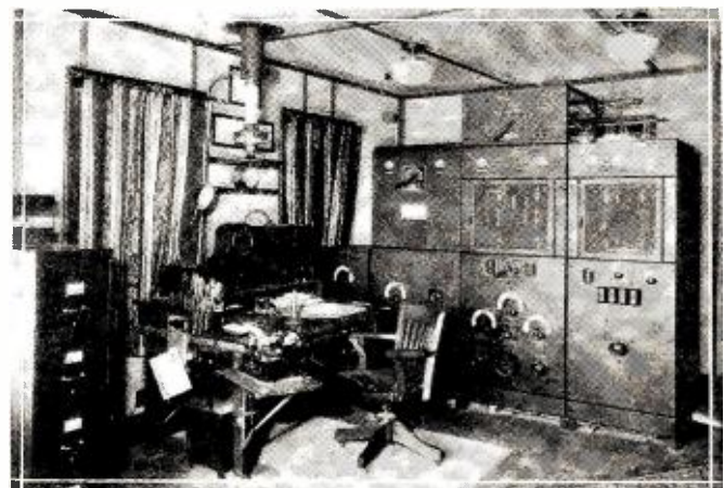
The above view is typical of the interior of the ground radio stations in the coast-to-coast communications network of the TAT-Maddux lines
