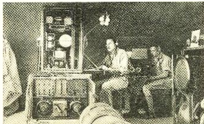
Above is an interior view of the station at Camp Hoover (Ochoa), February, 1930. The operators are First Class Privates, T. O. Cresnap and P. T. Peters
