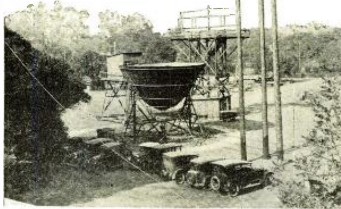
This is the chicken-wire reflector set up on the beach outside San Francisco Bay. It, too, swivels so that it may be aimed vertically or horizontally
