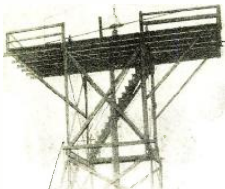
On this platform, atop a sixty-foot tower, all the field experiments in the measurement of the 4-meter beam transmission took place. The transmitter, located on a beach a few miles south of San Francisco Bay, was virtually aimed at this receiving target
