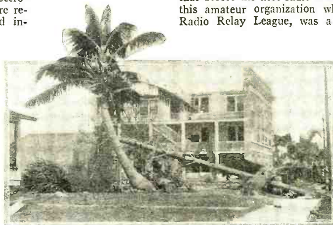
When the West Indian hurricane hit Florida, destroying the regular lines of communication, radio amateurs stepped into the breach and established contact with the outside world, aiding rescue work. The above Miami scene is typical of the widespread destruction
