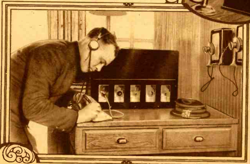
THE INTERIOR OF A RECEIVER. The dials are locked in the position for receiving on 526 meters, the wave-length of WNYC, and the front lid is locked, so that the set is ready at all times for emergencies. © Fotograms.
