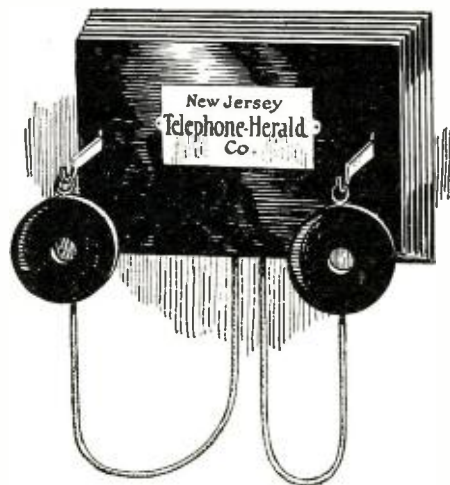
The subscriber's home installation was little more than a pair of receivers, as may be seen from the above sketch.
