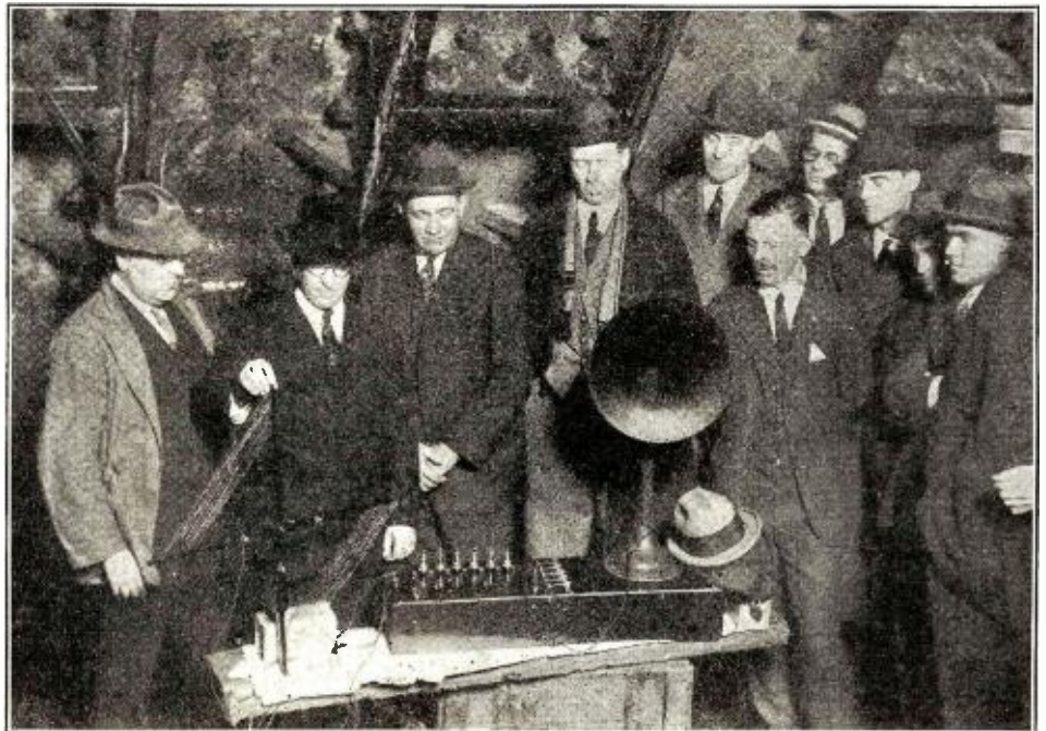
Photo of the assembly in the Hudson river tunnel during the test to determine the penetration of radio waves through the walls. A number of broadcast stations were successfully tuned in. © Photonews, N.Y.
