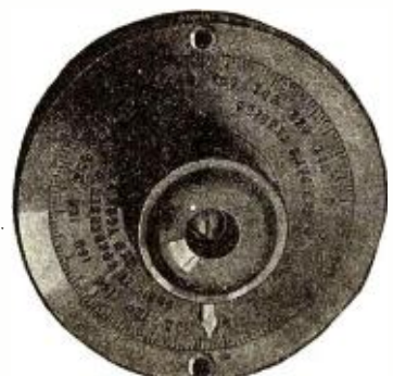
Fig. 11 Another type of compact mica variable condenser for receiving circuits.
