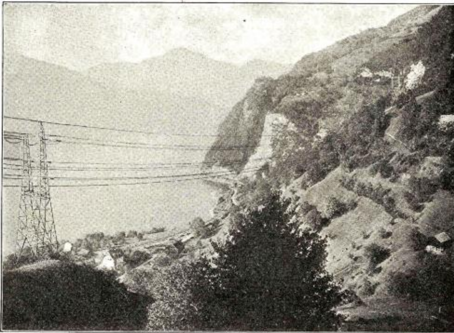
A 100,000-volt power line which is used, in the wired radio system, to guide the electromagnetic waves to the various sub-stations and permits instantaneous communication between any given stations.
