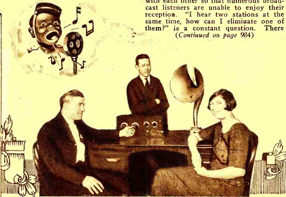
The Selectivity of a Receiver May Be Increased By Using a Short Aerial Such as Shown on the Left. It Becomes Easy Then, to Tune in Any Particular Station Without Interference.
