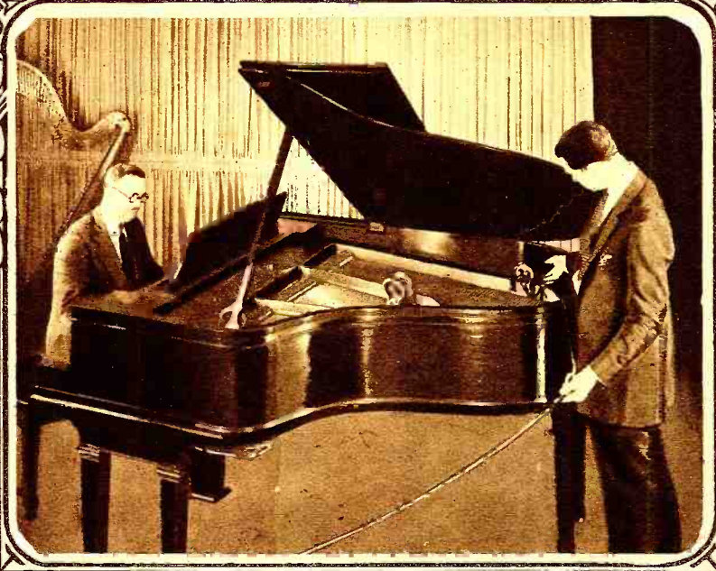
P. R. Fortin, of the Radio Department of the General Electric Company, Has Developed a Device Which Will Make the Piano Solo a Real Feature of a Broadcasting program at WGY. The Device, in Brief, Consists of a Magnet Between the Poles of Which is Pivoted a Suitable Coil System. The Magnet is Firmly Fastened to the Frame of the Piano and the Coil is Anchored to the Sound Board. By Means of This Pick-up Device All Tones in the Piano Are Faithfully Converted Into Corresponding Electric Currents Which Control the Radio Transmitter. When Heard on the Loud Speaker the Piano is No Longer a Twinkling Sound. The Listener Gets All the Characteristics of This Percussion Type of Instrument, the blow of the hammer, the singing tone and the Overtones.
