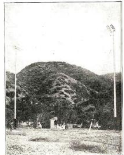
Fig. 2. The Transmitting Station at Avalon. The Receiving Loop is Fixt Up on the Other Small Cabin Which May Be Seen in the Background.
