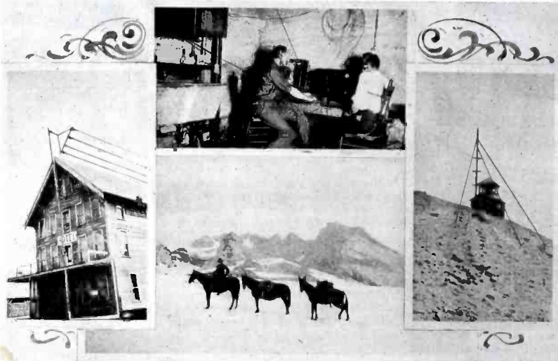
Left—Wireless Telephone Aerial at the Government Camp Hotel Mt. Hood. Upper Center—One of the Wireless Telephone Outfits Set Up for Experimenting in the Basement of Mr. Allen's Residence. Lower Center—Pack Horses Were Used in Transporting the Radiophone Sets Across Four Miles of Snow Covered Fields. Right—Great Difficulty Was Experienced in Erecting a Mast on the Mountain Top. The Lookout House Stands at an Elevation of 11,225 Feet.
