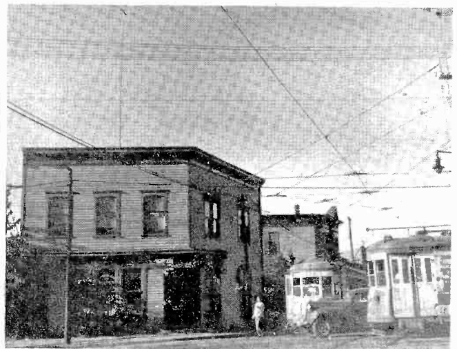
Trolley car, and auto interference was eliminated in this installation when the antenna was raised to 35 feet. At 15' and 25' the picture was unsatisfactory.
