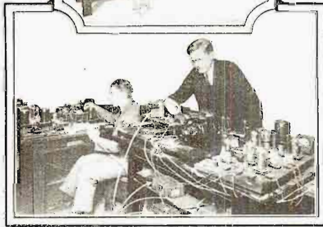
General view obtained through the courtesy of the Radio Corporation of America. Captain Richard Ranger of the R. C. A., inventor of the apparatus, is seen placing film upon drum of transmitter.
