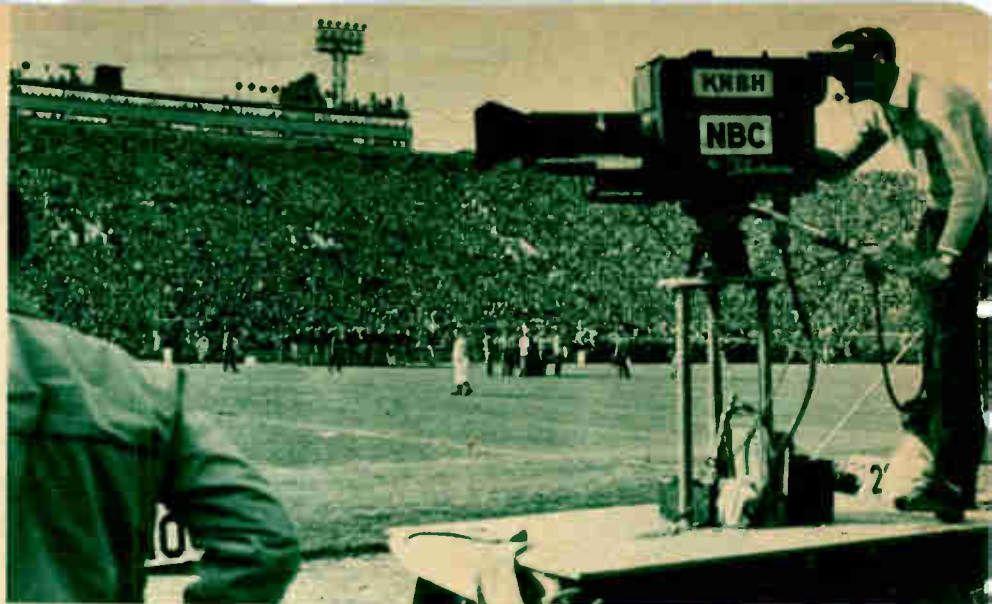
▲ JUST IN TIME FOR THE 1952 Rose Bowl classic between Illinois and Stanford Universities, KNBH came up with something new in the way of remote equipment. The "walkie-pushie" was used for the first time, and the mobile self-contained transmitter and camera moved right onto the field for close-ups. (NBC-Smith photo.)
