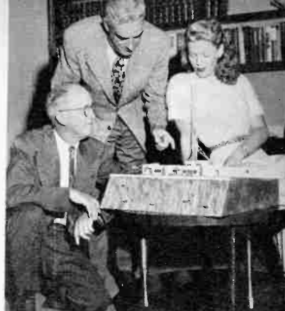
▲ LES BOWMAN , manager of things technical for CBS (center), Blake Compton, construction supervisor, and Shirley Christiansen look over a scale model of the building atop Mt. Wilson that houses both the KTV television and KNX-FM operations.
