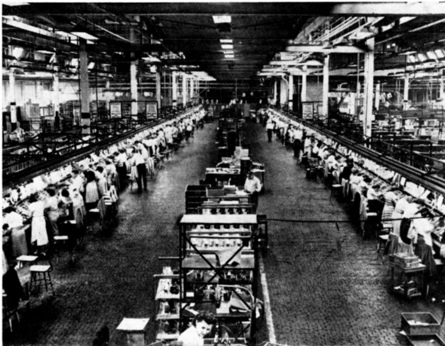
Two main television chassis assembly lines in the world's largest TV assembly plant. The Allen B. DuMont East Paterson plant spreads over 58 acres, nine and one-half of which is the main plant. Some 391,000 square feet of factory space make up the main plant. Bought for $1,350,000, conversion to TV assembly operations cost $750,000. At full capacity the plant will produce one TV receiver every 22 seconds.
