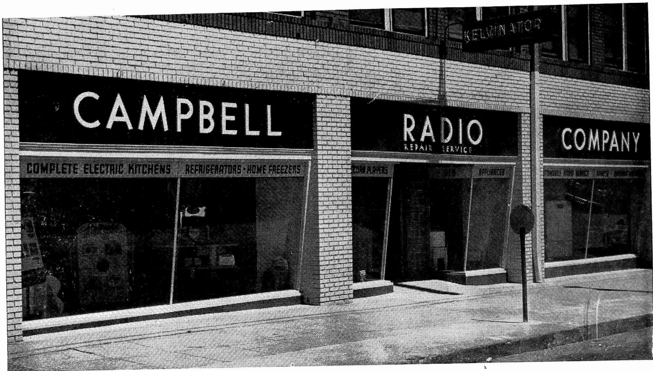
The remodeled front shows the slanting windows which are designed to eliminate glare at night.
