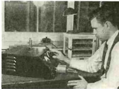
Measuring the losses in mica.
