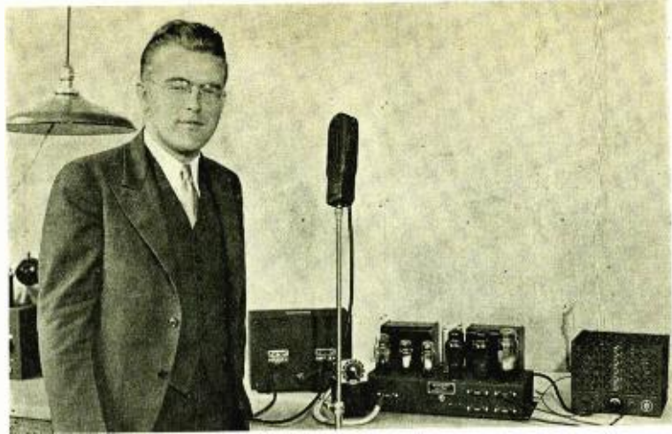
The author demonstrates the Lafayette Hi-Fidelity Amplifier described at length in the accompanying article. The ac-operated pre-amplifier was treated in an article in the October, 1934, issue of RADIO ENGINEERING.
