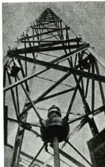
FIG. 3. LOOKING UP THROUGH THE LATTICE-WORK QUARTER-WAVE VERTICAL RADIATOR OF STATION WPFO
