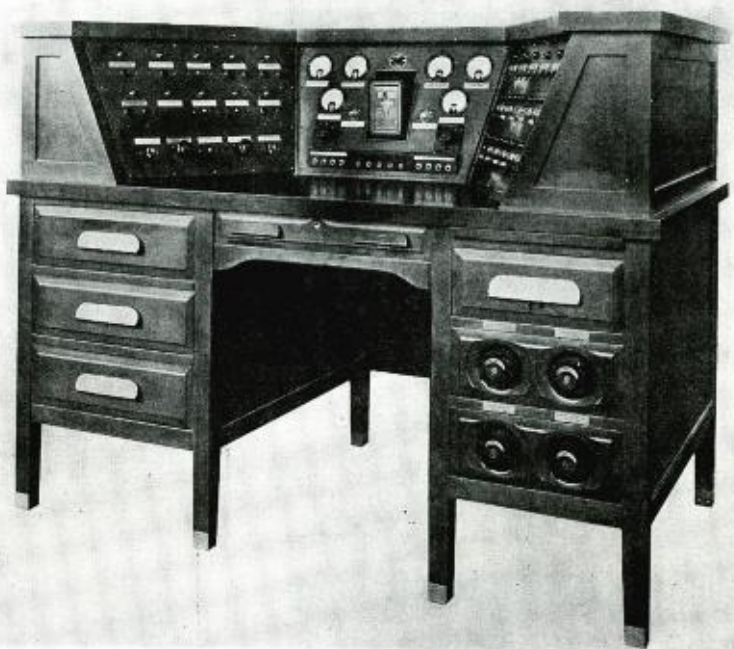
Thirty centrally located controls on the operator's control unit of WLW's new 500-kilowatt broadcast transmitter plant give complete automatic operation or any desired degree of manual control. The operation of the various circuits is indicated by 35 lights. The station, described in the January issue of RADIO ENGINEERING , was designed and built for the Crosley Radio Corporation by the RCA-Victor, Westinghouse and General Electric companies.
