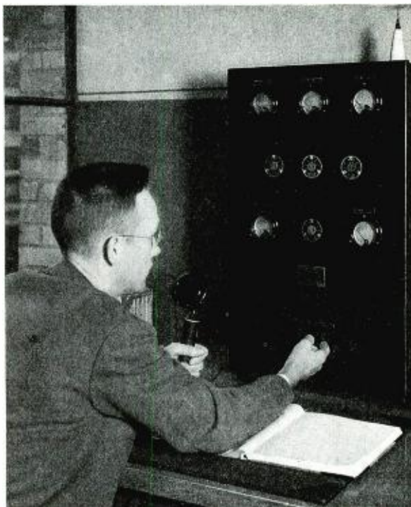
Operating Panel of Airport Ra- dio Transmitter
