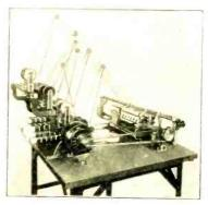
At the end of the layer, through a cam mechanism, together with a mercury switch, the glassine paper is automatically inserted in the winding, and the machine winds another layer over this paper and then the operation continues
