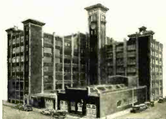
The huge Allen-Bradley plant at Milwaukee provides unlimited research and production facilities.
