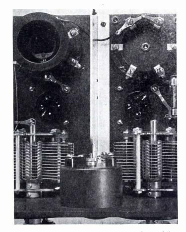
Details of the antenna and oscillator coll mountings, and the Interstage shielding. The center shield is cut away slightly to accommodate the voltmeter
