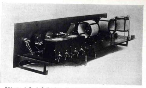
Rear view of the A. C. Aerodyne. The switch at the extreme left end of the panel is in the grid return lead of the detector, and changes this connection from negative to positive, according to the detector used
