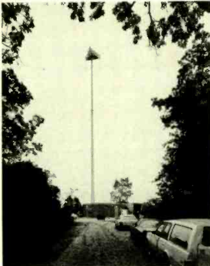
FIG. 1—CELL-SITE BUILDING is dwarfed by the 150-foot antenna tower. The two antennas below the platform are used for reception; the antenna above the platform is used for transmission.
