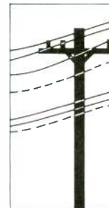
PRIMARY DISTRIBUTION LINES (4–35KV) 1–5μT, WITH MAGNETIC FIELD DROP OFF AT 1/r^2
