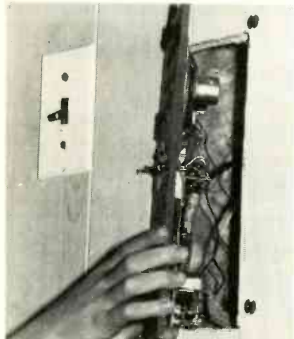
FIG. 4—CIRCUIT BOARD, speaker, and switch are set into wall on a piece of paneling, near a wall switch to connect to house ground.
