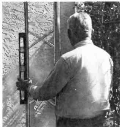
FIG. 6—CHECK FOR VERTICAL orientation with a spirit level or a plumbline.
