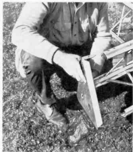
FIG. 3—BOLTING THE BASEPLATE to the legs of the tower.
