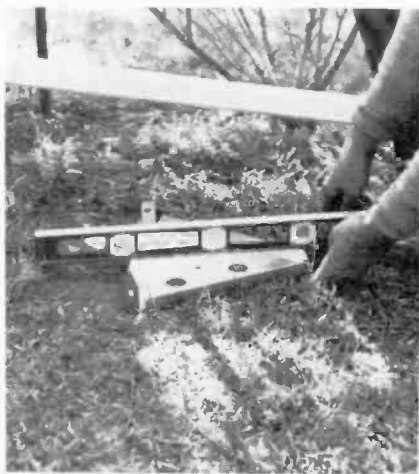
FIG. 1—LEVELING THE BASEPLATE makes a good foundation for the whole job.
