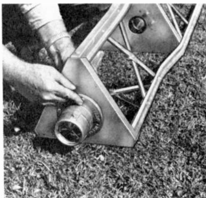
FIG. 8—THE TOWER'S TOP SECTION is equipped to hold a rotator, if needed.
