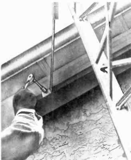
FIG. 5—BRACKET MUST BE FASTENED securely to a solid part of the house.
