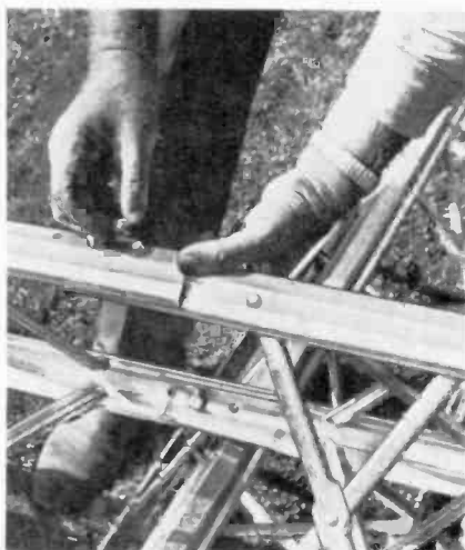
FIG. 2—SECTIONS ARE FASTENED, preferably on the ground before raising.
