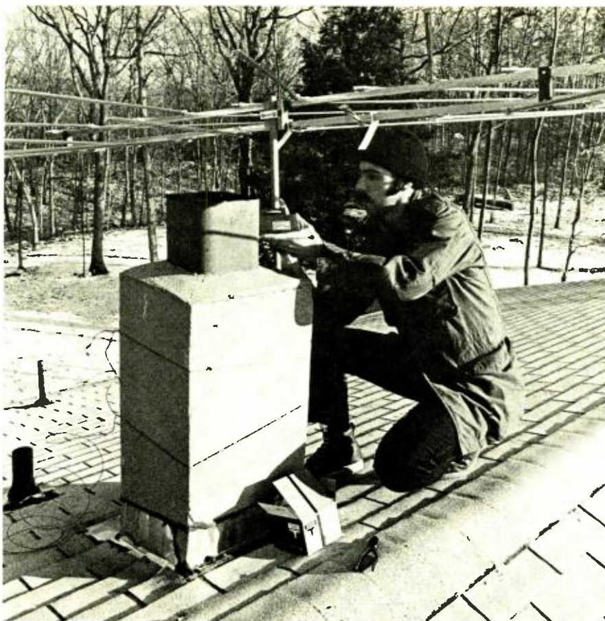
BOOSTER MOUNTS ON MAST and connects between lead in and transmission coax. In typical installations the antenna should be mounted further above the chimney.
