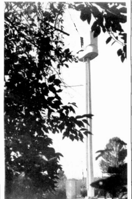
THESE MODERNISTIC CANISTERS will house seven bi-directional transmitter and receiver systems, plus a standby, together with antennas and interconnecting equipment.
