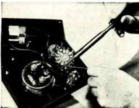
Construction of Multimeter.
