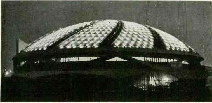
G-E hostess points out control panel of "Directo-Matic" apparatus (right) used to control spectacular night-time dome lighting at G-E pavilion (above). Crisscross roof-supporting grid of steel tubes is flooded with 2,112 colored lights dimmed and turned on and off by silicon controlled rectifiers. Reels at right carry punched paper tape that controls lights.
