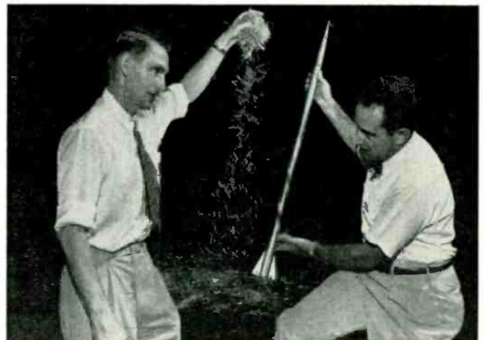
Fig. 8—High-frequency chaff which is dispensed by small rockets. U. S. Army
