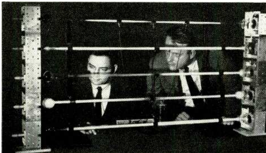
Kumar Patel and William Bennett, Jr., of Bell Laboratories, with their five new optical masers, containing helium, neon, argon, krypton and xenon. These masers, though fitted for dc excitation, are being excited by rf (transmitted through the clip type capacitors) in this experiment.
