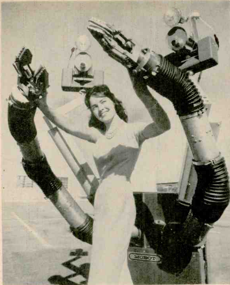
SCIENCE-FICTION MONSTER substitutes for man in dangerous places. Two TV camera eyes transmit pictures of its handiwork to human operator at a remote-control console. They can be remotely adjusted to view any action of the robot. Arms of the Hughes Aircraft Robot are double-jointed at shoulders, elbows and wrists for extreme flexibility.
