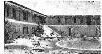
APARTMENT—39 Outlets—One Antenna—No Amplification: The Del Rio—10236 Old River School Road, Downey, Calif.
