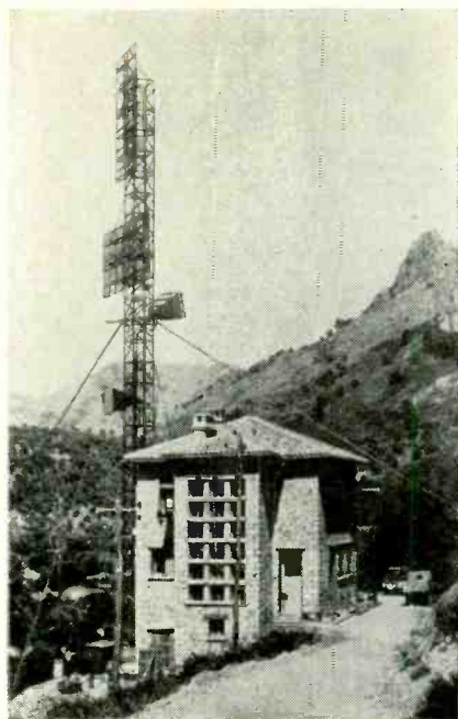
Compagnie Générale de TSF microwave installation at Calenza in Corsica.
