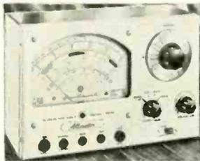
per volt): 0-15, 75, 150, 300, 750, 1,500, 7,500; 3 resistance ranges: 0-2,000, 200,000 ohms, 20 megohms, 2 capacitance ranges: .00025-0.3  $\mu$ f, .05-30  $\mu$ f, 5 dc current ranges: 0-75  $\mu$ amp; 0-7.5, 75, 750 ma; 0-15 amps; 3 decibel ranges, -6 +18, 14-38, 34-58. Superior Instrument Co., 2435 White Plains Rd., New York 67, N. Y.
