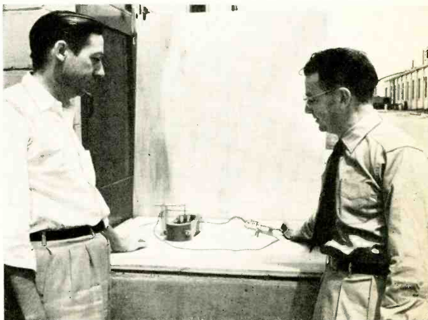
Donald C. Reynolds (left) and Lt. Colonel Gerard M. Leies observe the solar generator as it turns small direct-current motor at 73 revolutions per minute.
