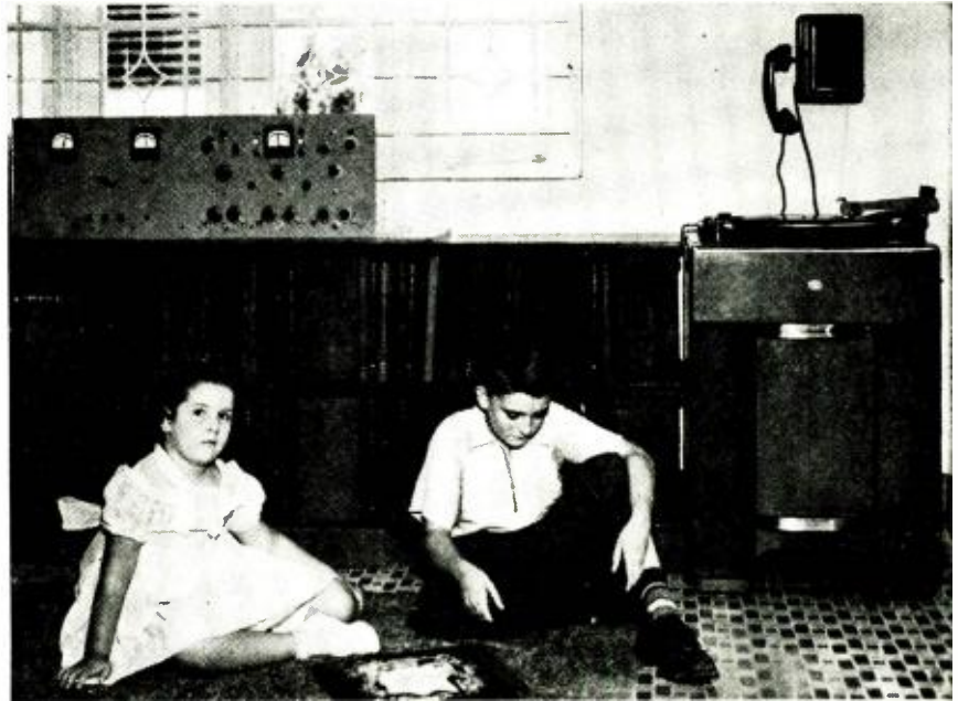
Home Installation showing professional appearance of the Rico amplifier
