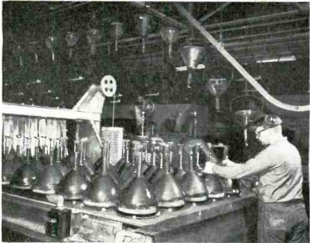
After coating and screening, the bulbs go through a high-temperature oven to drive out all organic matter. The operator above takes the bulbs from the conveyor as they emerge from the oven and puts them on the overhead conveyer which takes them on to the next step.
