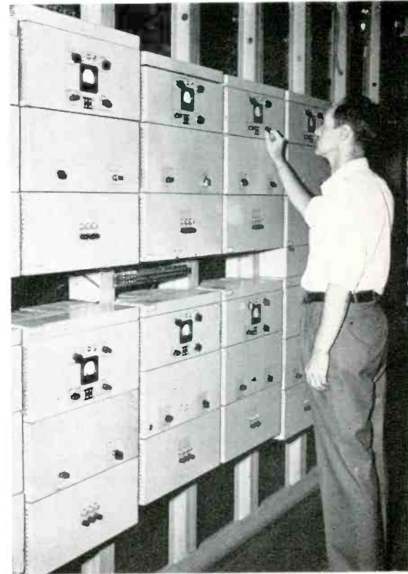
Carrier equipment panels as now used on railroad wire line circuits which can be modified for microwave applications.
