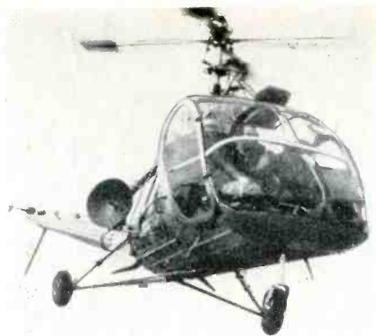
Airborne helicopter for use in aerial surveys. Note receiving parabola.
