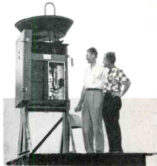
Remote-type r.f. unit at base of water tank at Grande Ecaille.
