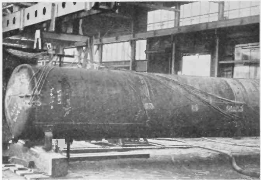
Typical strain gauge installation on a boiler to determine stresses.
