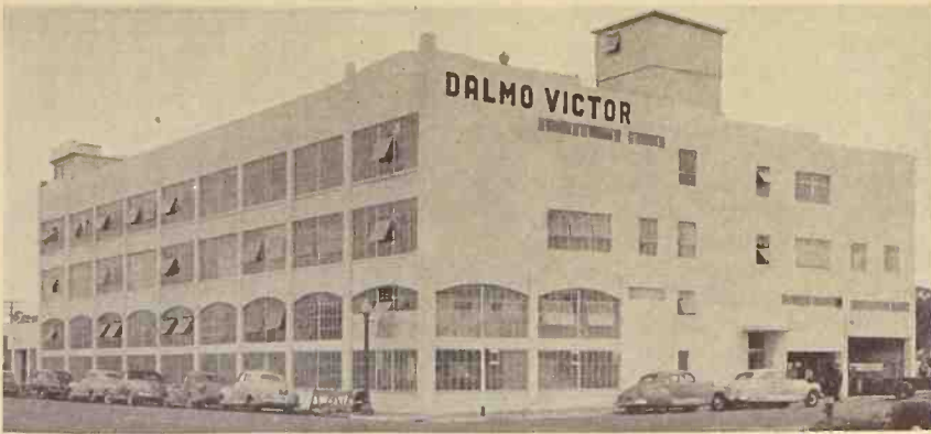
Fig. 4. Antenna pattern penthouse test shacks atop the Dalmo Victor plant.
