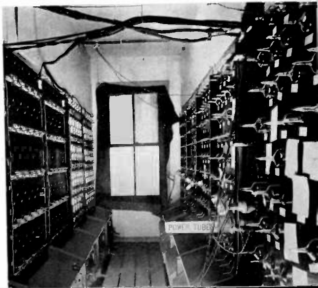
Figure 2—Power amplifier of the Arlington, Virginia, experimental transmitter, 1915.
