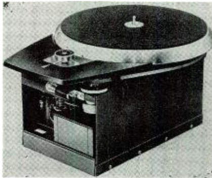
New at the institute of High Fidelity Manufacturers 1957 Chicago Music and High Fidelity Show, Sept. 17-21, will be this completely electronically driven turntable manufactured by Fairchild Recording Equipment Co. Four speeds are selected by feeding a hysteresis motor with specific frequencies supplied from a self-contained variable signal generator.
