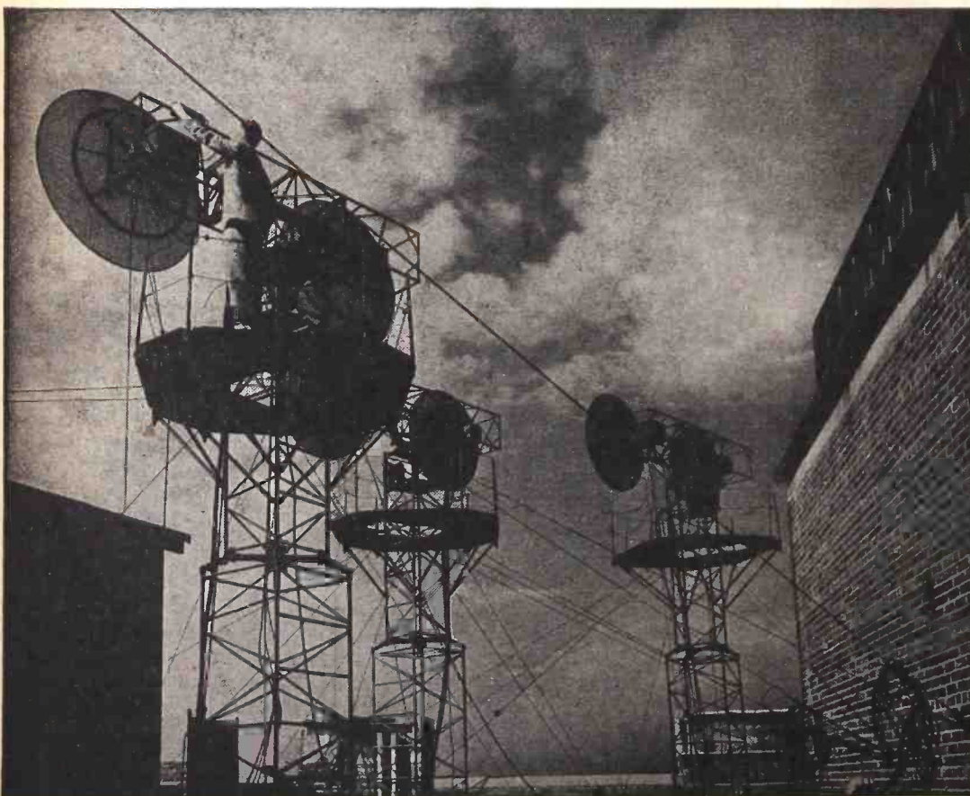
Rear view of three parabolic antennas on roof of the Telephone Building, New York City.
