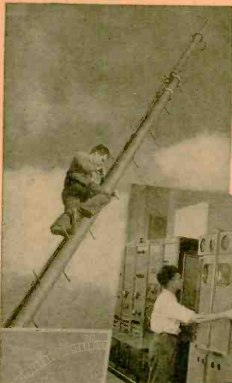
Below: The 10,000-watt transmitter of W7INY, Frequency Modulation station of WOR, New York. The transmitting plant is located at 444 Madison Avenue, New York City.
