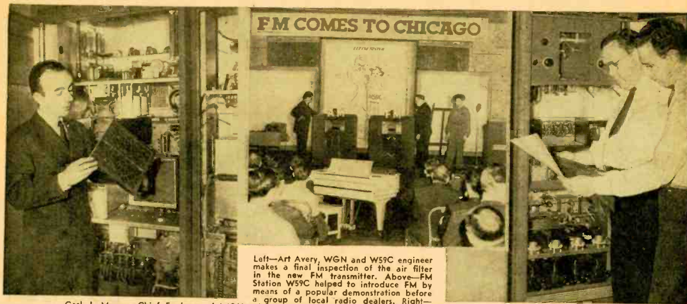
Left—Art Avery, WGN and W59C engineer makes a final inspection of the air filter in the new FM transmitter. Above—FM Station W59C helped to introduce FM by means of a popular demonstration before a group of local radio dealers. Right—Carl J. Meyers, Chief Engineer of WGN and W59C (left) and his Assistant, Clyde White, during installation of FM transmitter.
